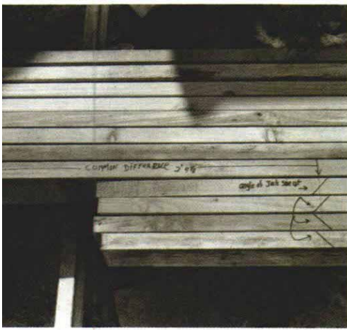
Jack rafters stacked on a rafter bench show the common difference of 2 ft. 4 7 / 8 in. on an 8-in-12 pitch using a 24-in. spacing. The diagonal lines indicate the direction of the side cut that will produce pairs of jacks (left and right) for each hip rafter. The bird's mouth and tail will be marked with the common-rafter layout tee.
